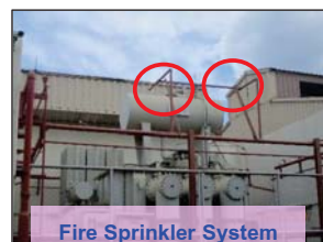
Fire Sprinkler System
